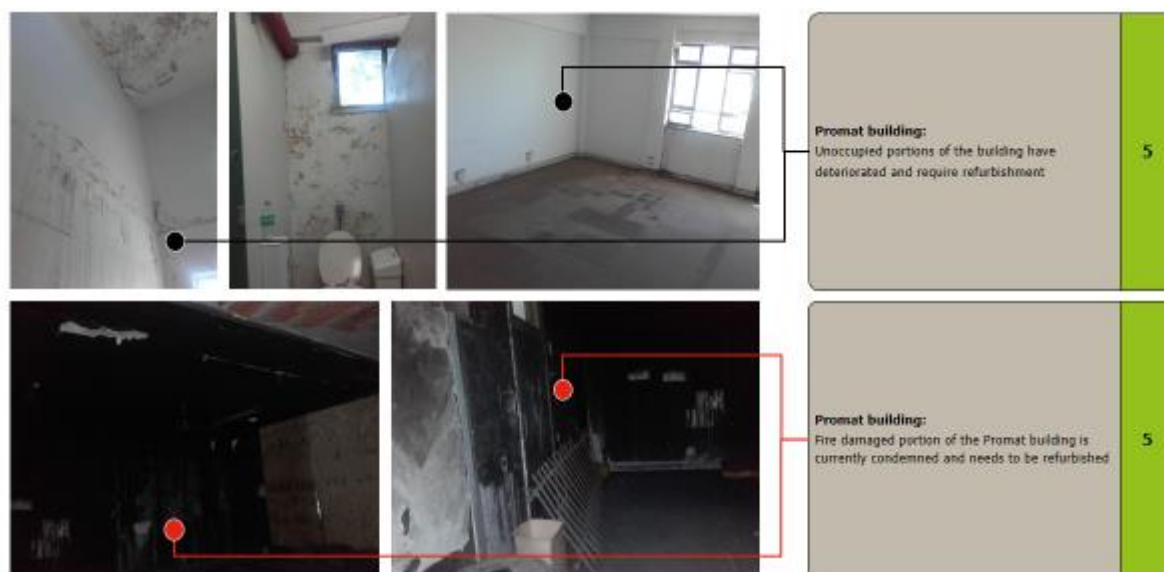
Fig 4. Promat Building burnt room, damp walls and roof slab
